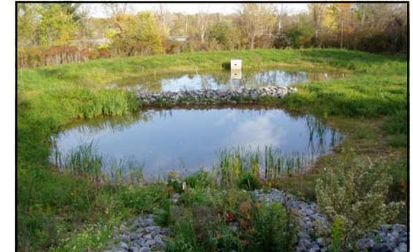
Stormwater retention ponds provide effective water quality control by using forebays for sediment settling, and have controlled-discharge outlets for flood control.
