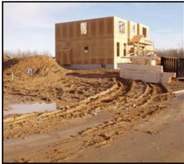
Rain could easily wash this loose soil into the storm sewer and into a nearby stream, causing a water quality standards violation that could cost the site operator up to \$37,500 each day it occurs.
